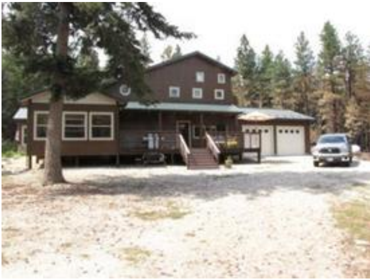
Figure 1: Residence did not have any burnable vegetation near the house. The deck had rock underneath the composite decking. It had a metal roof and cement board siding and a gravel driveway surrounded the house on two sides. Trees were cleared away from the house.
