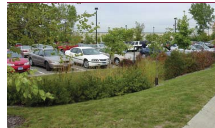
A bioretention cell manages runoff from the imperviousness of a commercial parking lot. A bioretention cell is a low impact development practice because it allows rainwater to infiltrate, minimizes flooding and protects water quality.
