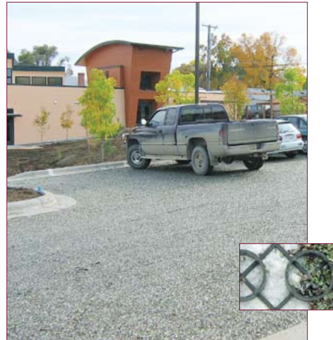
The parking lot of the Northern Plains Resource Council building in Billings, Montana consists of a grid of rings (recycled plastic) over a geotextile fabric that holds the small gravels in place. 100% recycled glass cullet was used instead of gravel in the top layer.
