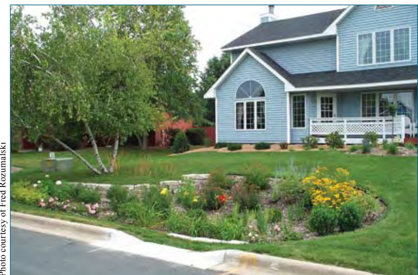
This rain garden is strategically placed to capture runoff from the lawn and street. Rain gardens can also be designed to capture roof and sidewalk runoff.
